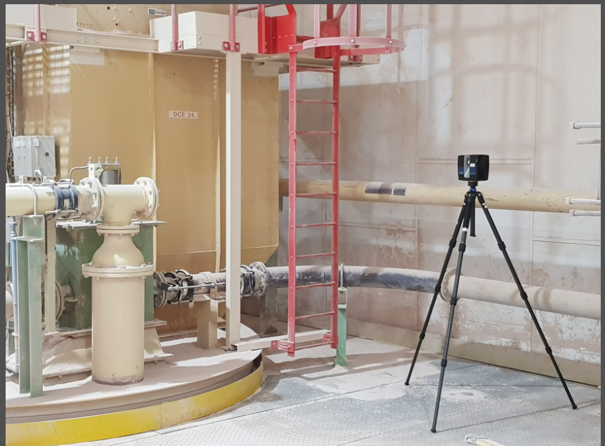
modern 3D laser scanner set-up and in position on site
